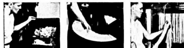
ANOTHER PERFECT TEST RUN. Here, R. C. Benson, Durum Department, checks extrusion from the hydraulic press, a part of the miniature spaghetti plant in operation at Pillsbury's fully-equipped Products Control Laboratory. Capacity of the plant is 20 pounds per hour.
